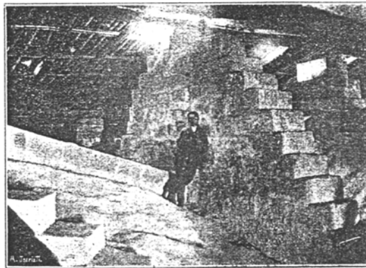
Figure 24 : Weights over the central keystone of Palma de Mallorca (Rubiò, 1912) and transverse arches (Rubiò, 1912)
